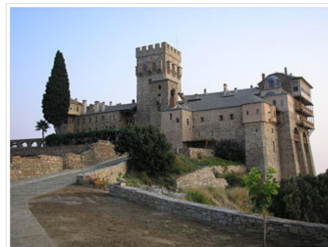
Stavronikita monastery, Mount Athos, Greece (South-East view)
