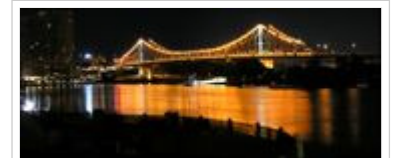
The Story Bridge in Brisbane, Australia, built in 1940 with modern materials, is an example of a steel cantilever bridge.
