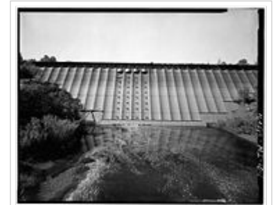
Red Ridge steel dam, b. 1905, Michigan.
