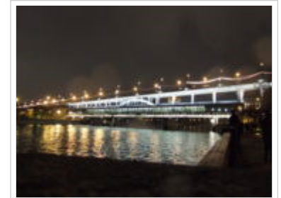
"Metrobridge" Vorobyovy Gory ( ru:Метропонтон) double-deck bridge in Moscow carries the Moscow Metro.
