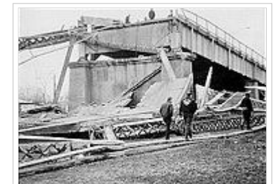
The collapsed Silver Bridge, as seen from the Ohio side
