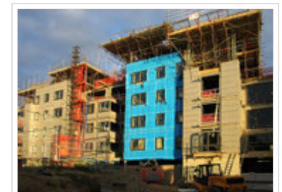
Building construction for several apartment blocks
