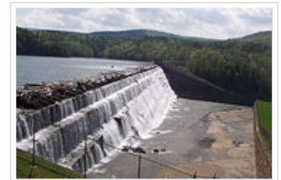
The Gilboa Dam in the Catskill Mountains of New York State is an example of a "solid" gravity dam.
