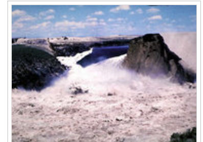
The reservoir emptying through the failed Teton Dam.
