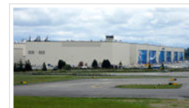
Boeing's Everett facility, selected as the site of 787 final assembly.
