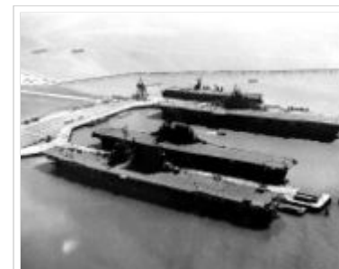
4 US Navy carriers right after the war, showing the size and length difference between an early battlecruiser conversion, the Saratoga (bottom), an early fleet carrier Enterprise (2nd from bottom), a war time built Essex -class carrier (2nd from top, the Hornet ) and a light carrier based on a cruiser hull, the San Jacinto (top).
