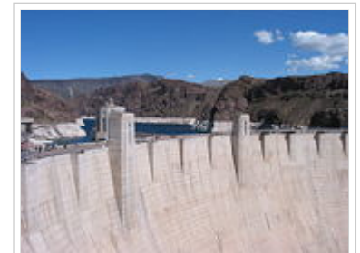
Hoover Dam, a concrete arch-gravity dam in the Black Canyon of the Colorado River.
