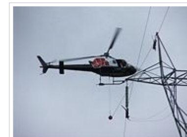
A-Star pulling rope through skywire traveller
