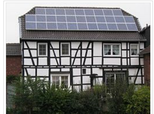
Timber framed house with a photovoltaic array
