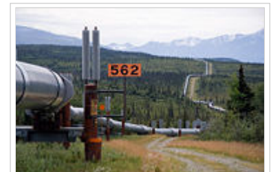
Trans-Alaska Pipeline for crude oil.
