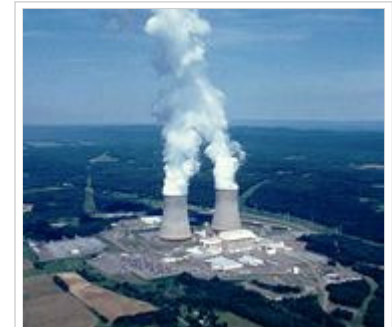
The Susquehanna Steam Electric Station, a boiling water reactor. The nuclear reactors are located inside the rectangular containment buildings towards the front of the cooling towers. The towers in the background vent water vapor.
