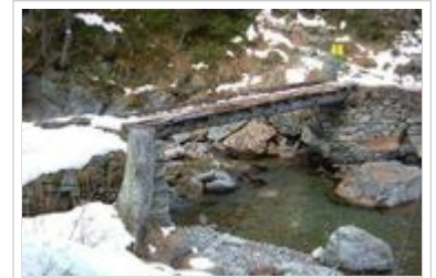
A log bridge in the French Alps near Vallorcine.
