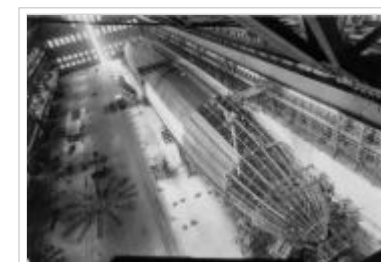
Construction of the USS Shenandoah (ZR-1), 1923
