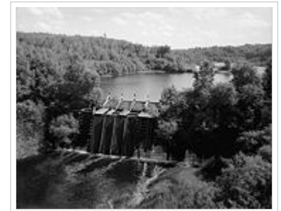
A timber crib dam in Michigan, photographed in 1978.
