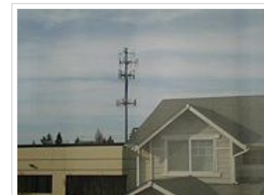
Cell Phone tower located in Lynnwood, WA.
