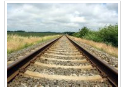
Concrete ties (sleepers)
