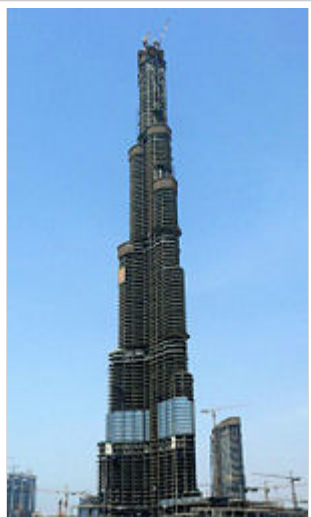
Burj Dubai, the world's tallest building, currently under construction in Dubai
