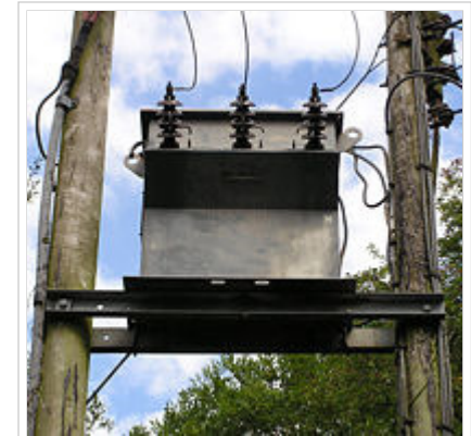
Electrical Engineers design complex power systems...
