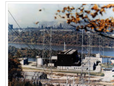
The Shippingport Atomic Power Station in Shippingport, Pennsylvania was the first commercial reactor in the USA and was opened in 1957.
