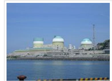
The Ikata Nuclear Power Plant, a pressurized water reactor that has no cooling tower, but cools by direct exchange with the ocean.
