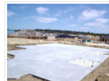
A slab-on-grade foundation
