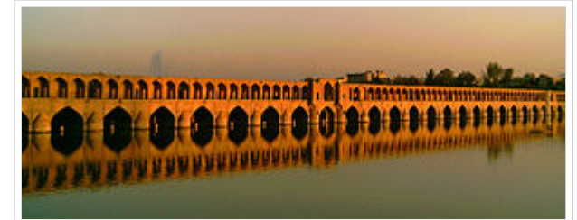
The masonry Bridge of 33 Arches over the Zayandeh River is the epitome of Safavid dynasty (1502-1722) bridge design. Esfahan, Iran.
