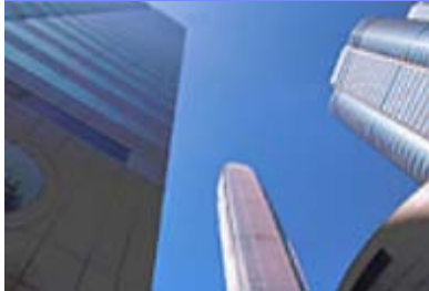
Real Estate and Facilities
