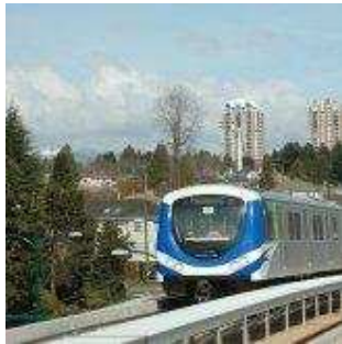
Signalling systems for urban transport networks.
