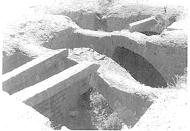
Fig. 20. Early Byzantine domestic cistern roofed with slabs carried on arched rib walls, at Androna (al-Andarin), Syria. Photo: A. Wilson.
